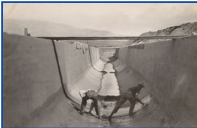
Lining the conduit in Mojave Division. Oct. 1908. Photo by J. B. Lippincott. Joseph B. Lippincott Collection; LIPP Box 78, no. 304.
